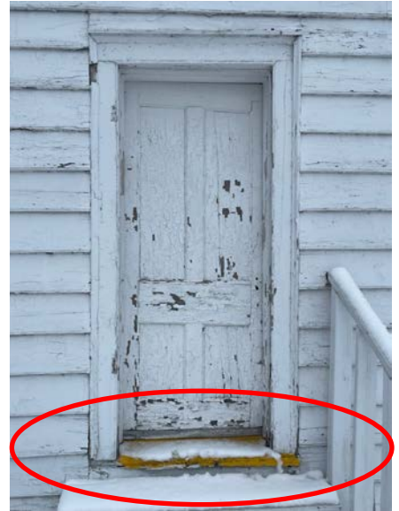
Area of rot to address and door to repair or replace
