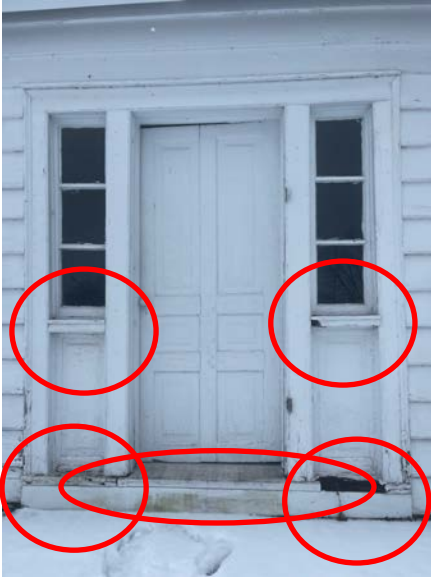
Areas of rot to address on North side
