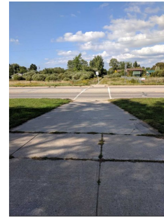
Concern: Sidewalk leads to a narrow footpath inaccessible to wheelchairs (Marquette)
