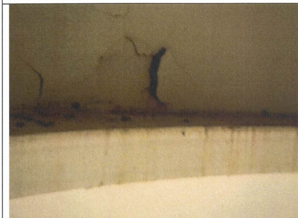
Lifting at pedestal stiffener ring
