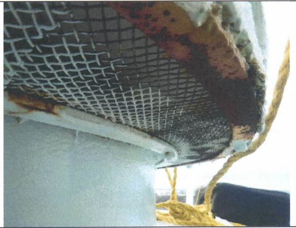
Access tube vent screen and bands
