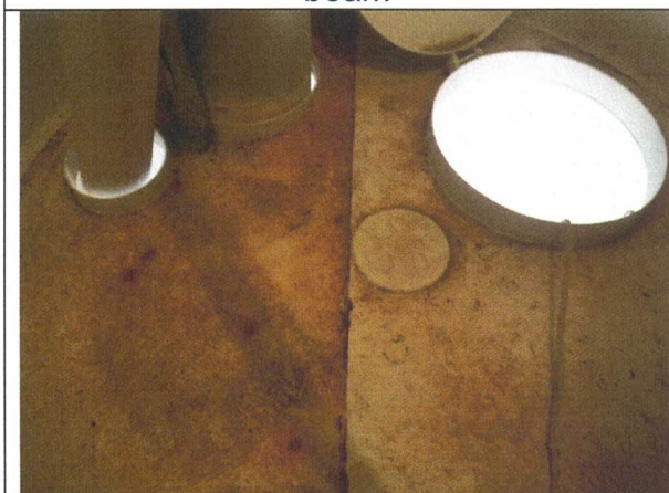
Corrosion on condensate platform
