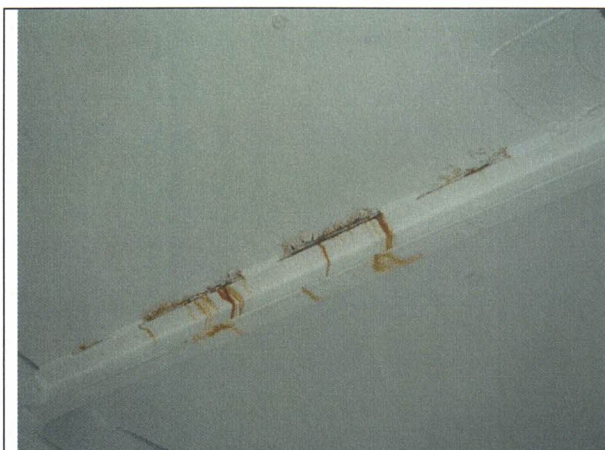
Corrosion at condensate platform support beam
