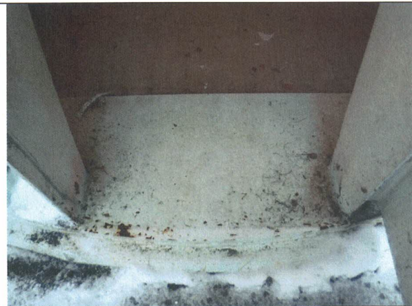
Minor coating breaks at basebell entrance
