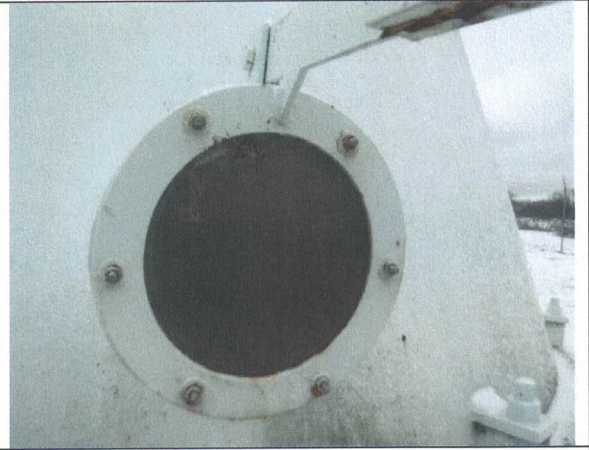
Overflow pipe flap gate with 24-mesh screen
