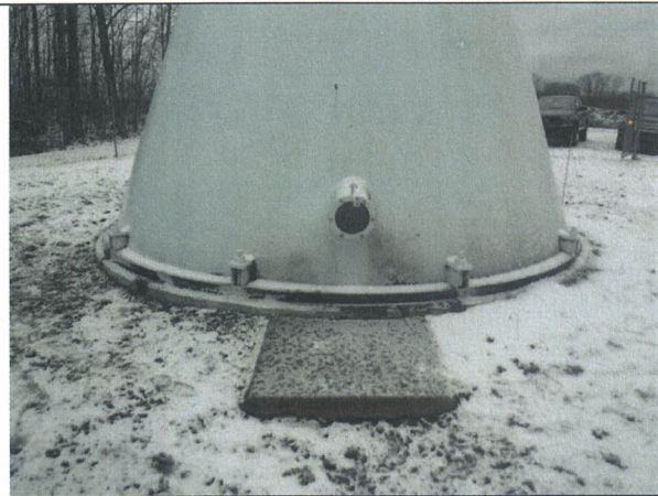
Overflow pipe and splash pad
