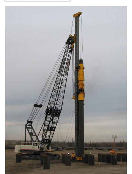
Sheet pile driving with a diesel impact hammer
